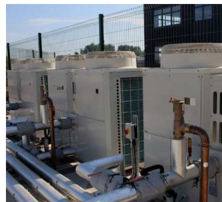
Roof Mounted ASHP Cascade
