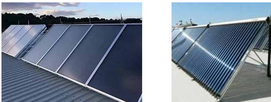
Figure 7 - Flat Plate (Left) and Evacuated Tube (Right) Solar Thermal Panels
