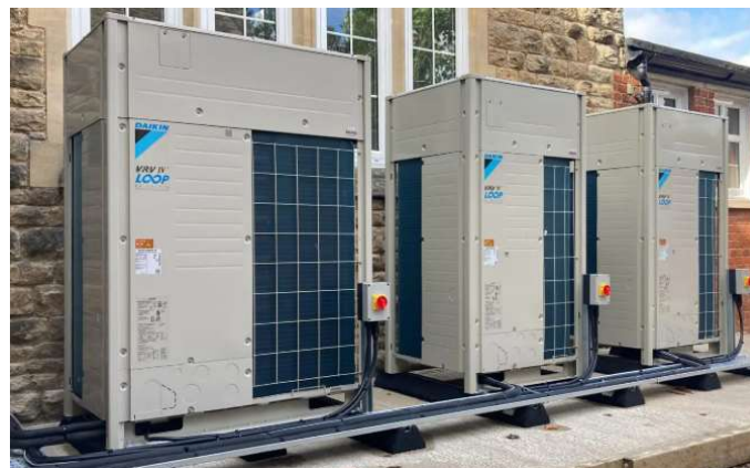
Figure 9 - Image above showing a typical VRF (VRV) Air Conditioning System
